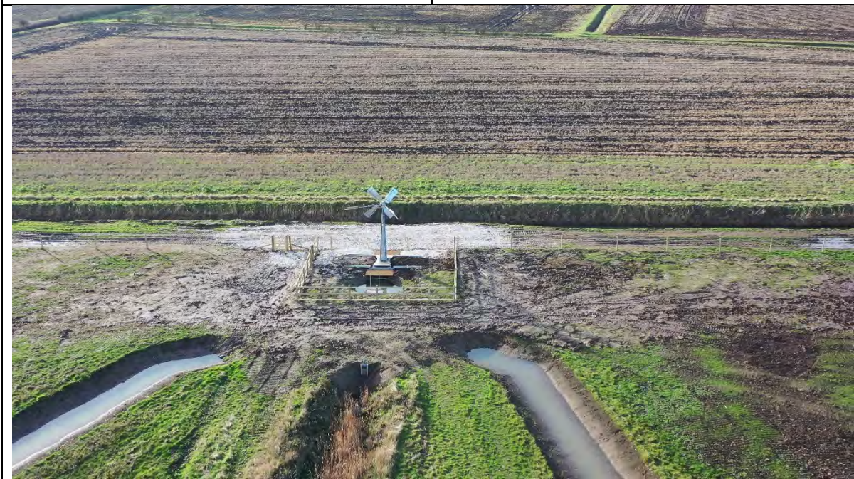
Figure 5c – Wind Pump abstracting water from Halton Drain
