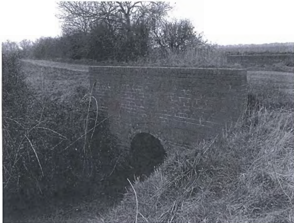
Photograph 1: Culvert connecting East Halton Drain (foreground) to East Halton Beck
